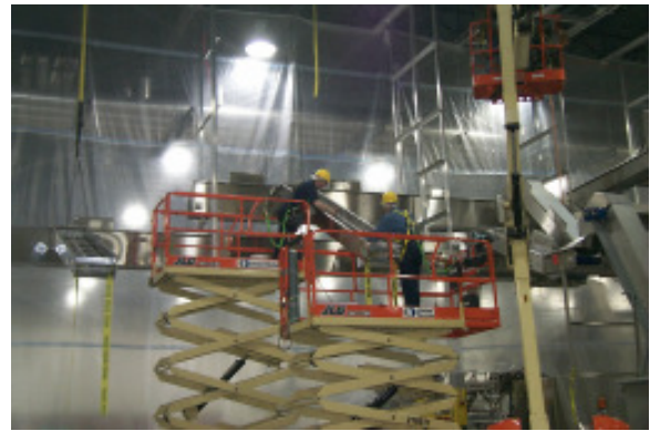
KLEENLine Installation Crew
